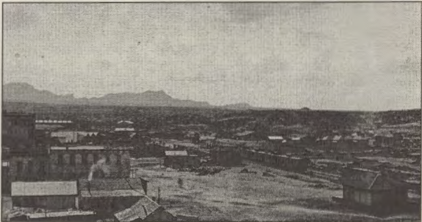
Looking from the Pierson Hotel toward Sunset Heights, note the main train line
