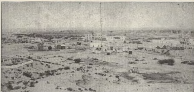
1882 from the area of Mesa Gardens looking to downtown, note the railroad tracks
