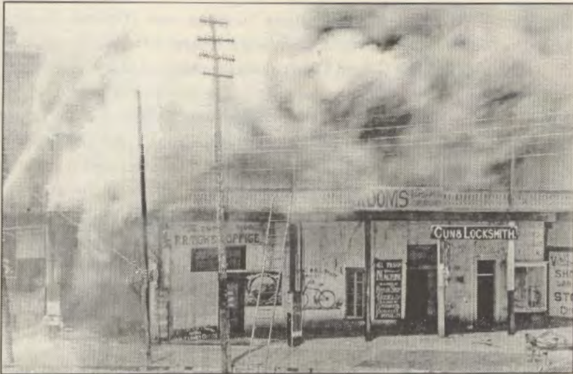
The Central Hotel Fire
